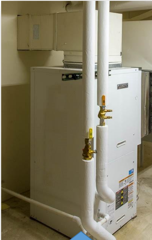
Vertical GHP (water-to-air GHP)
