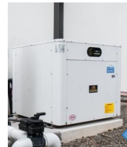
Horizontal; GHP (water-to-air GHP)
