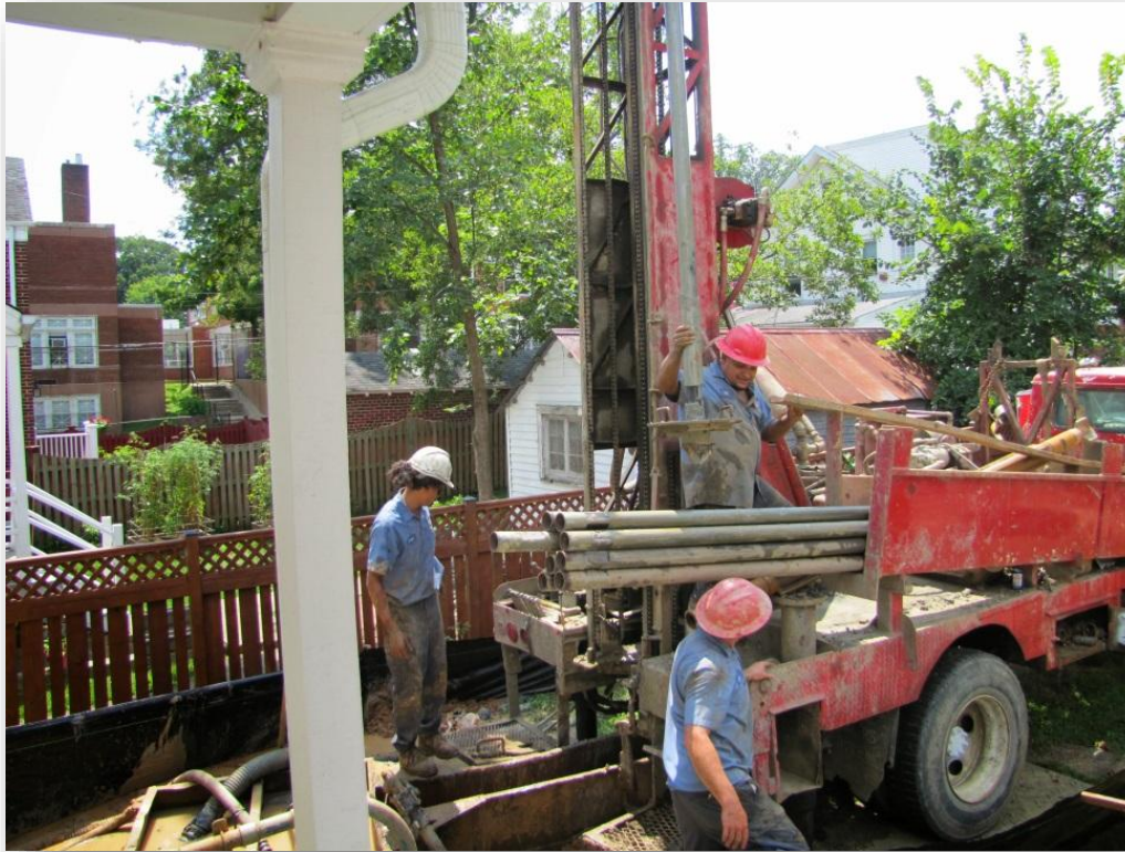
Vertical Closed Loops (tight spot)
