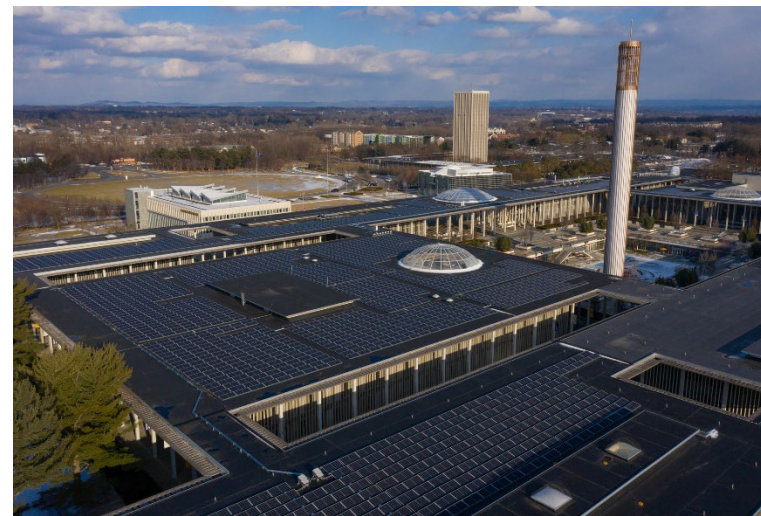
1.9 MW rooftop solar PV
