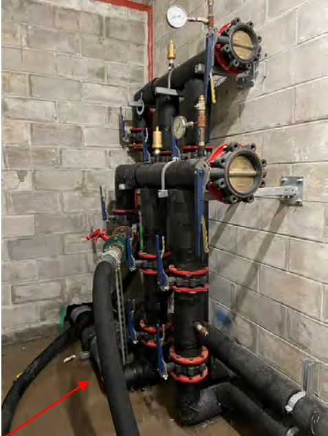
Purging & flushing to remove air and debris in loops
