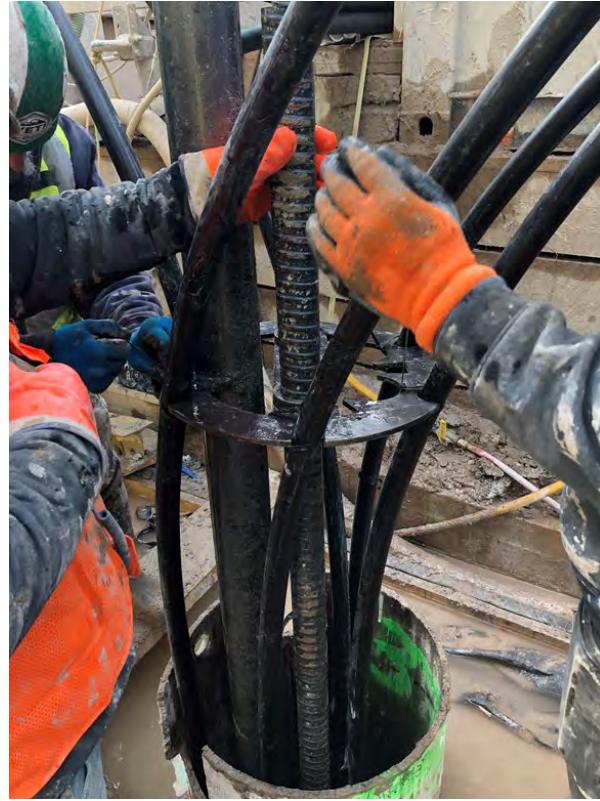
Loops equally spaced around circumference
