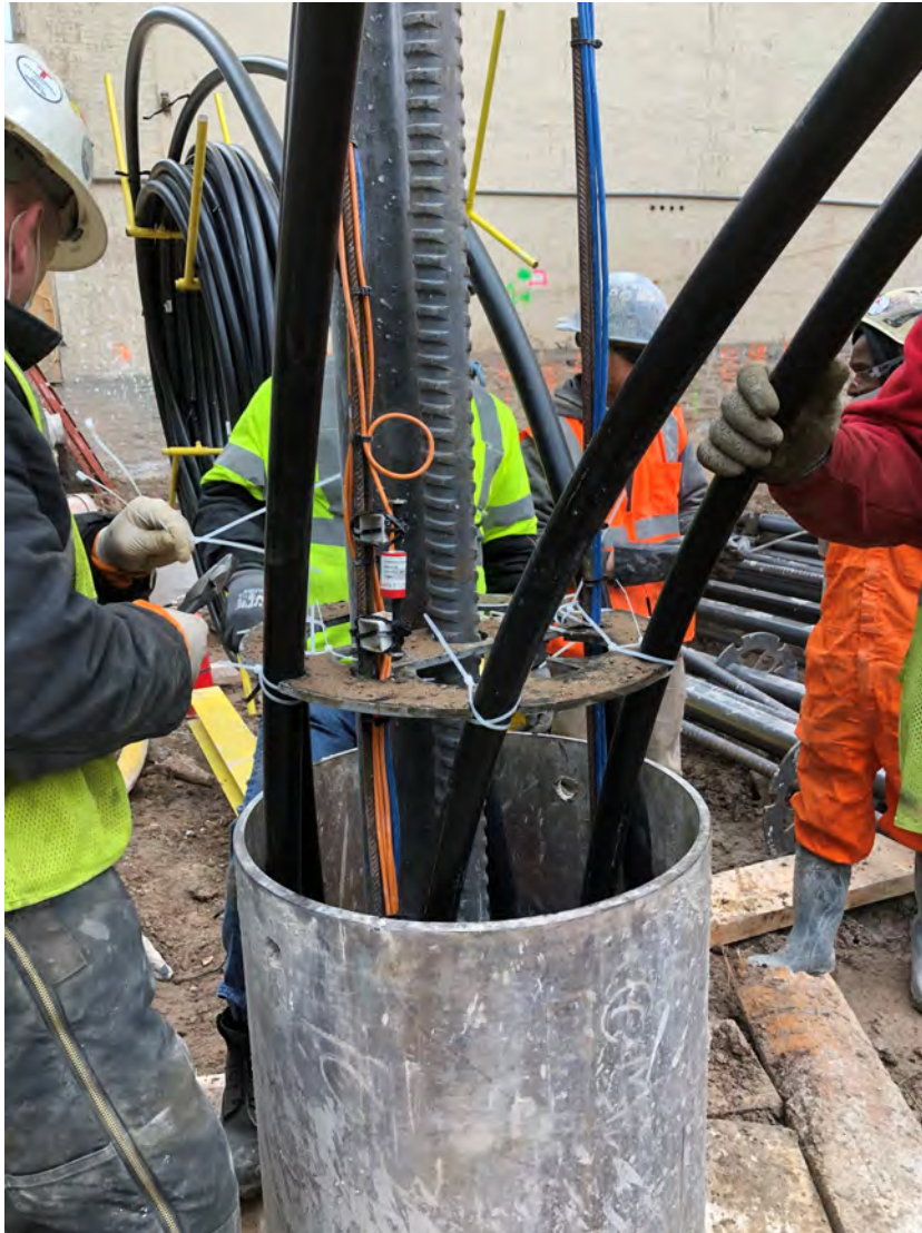
Pile 4A & 10C - 20VW & 14 Temperature sensors (Pile 10C Conductivity test pile) Pile 6 Mini – 14VW sensors Instrumentation positioned at 2, 5, 10, 15, 20, 30, 40, 50, 60, 70, 80, 90, 95, 98 ft below pile cut off
