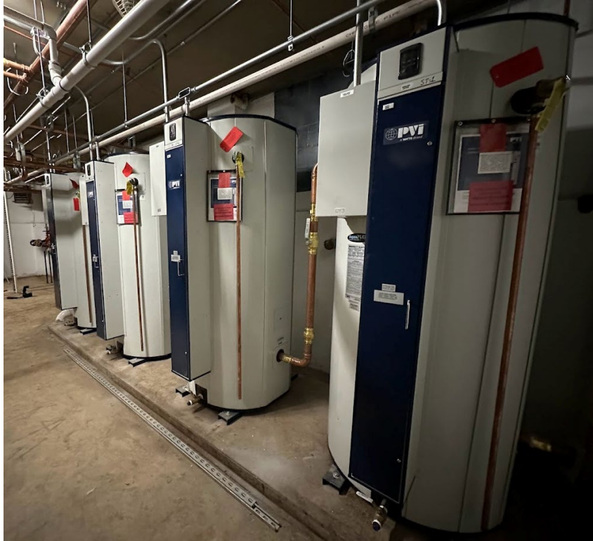
Domestic Hot Water Storage Tanks
