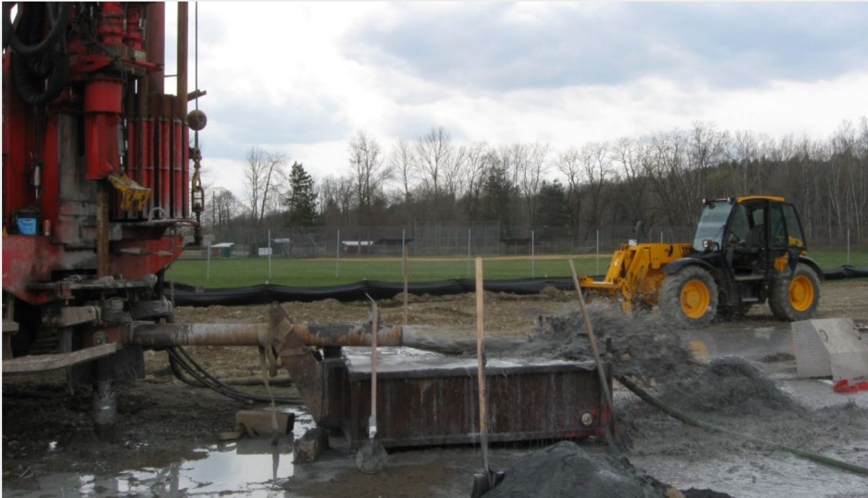
Methane gas unloading of borehole Q1 Discharged ~100 gal/min of saline water for 15 minutes
