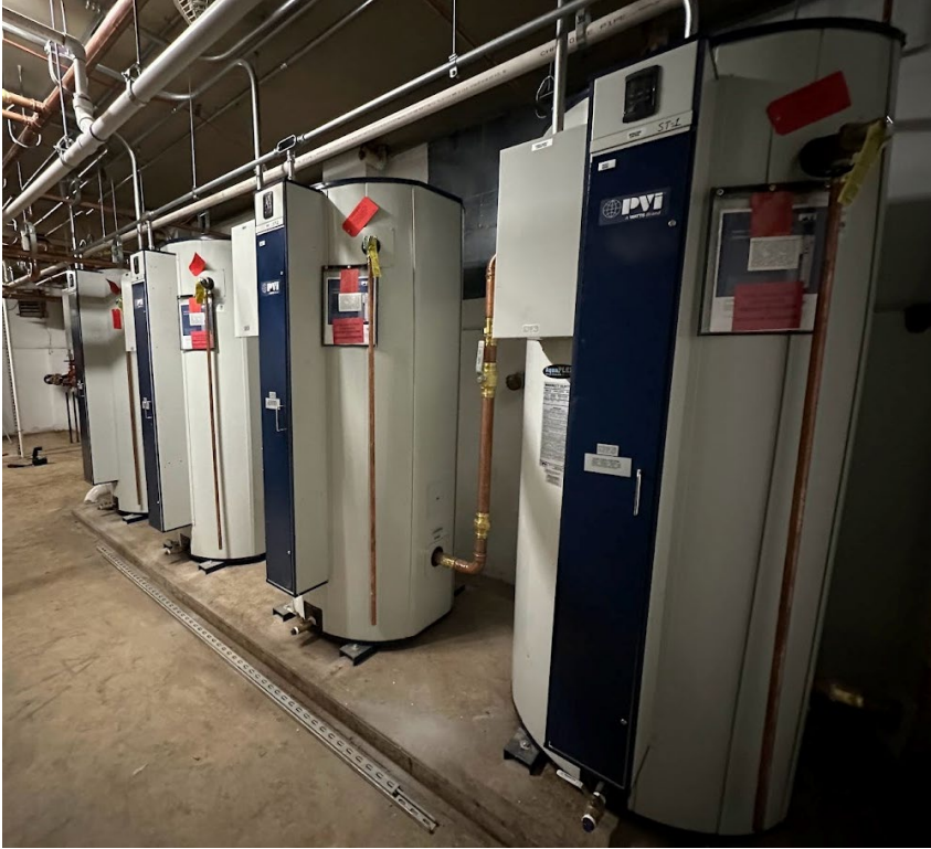
Domestic Hot Water Storage Tanks
