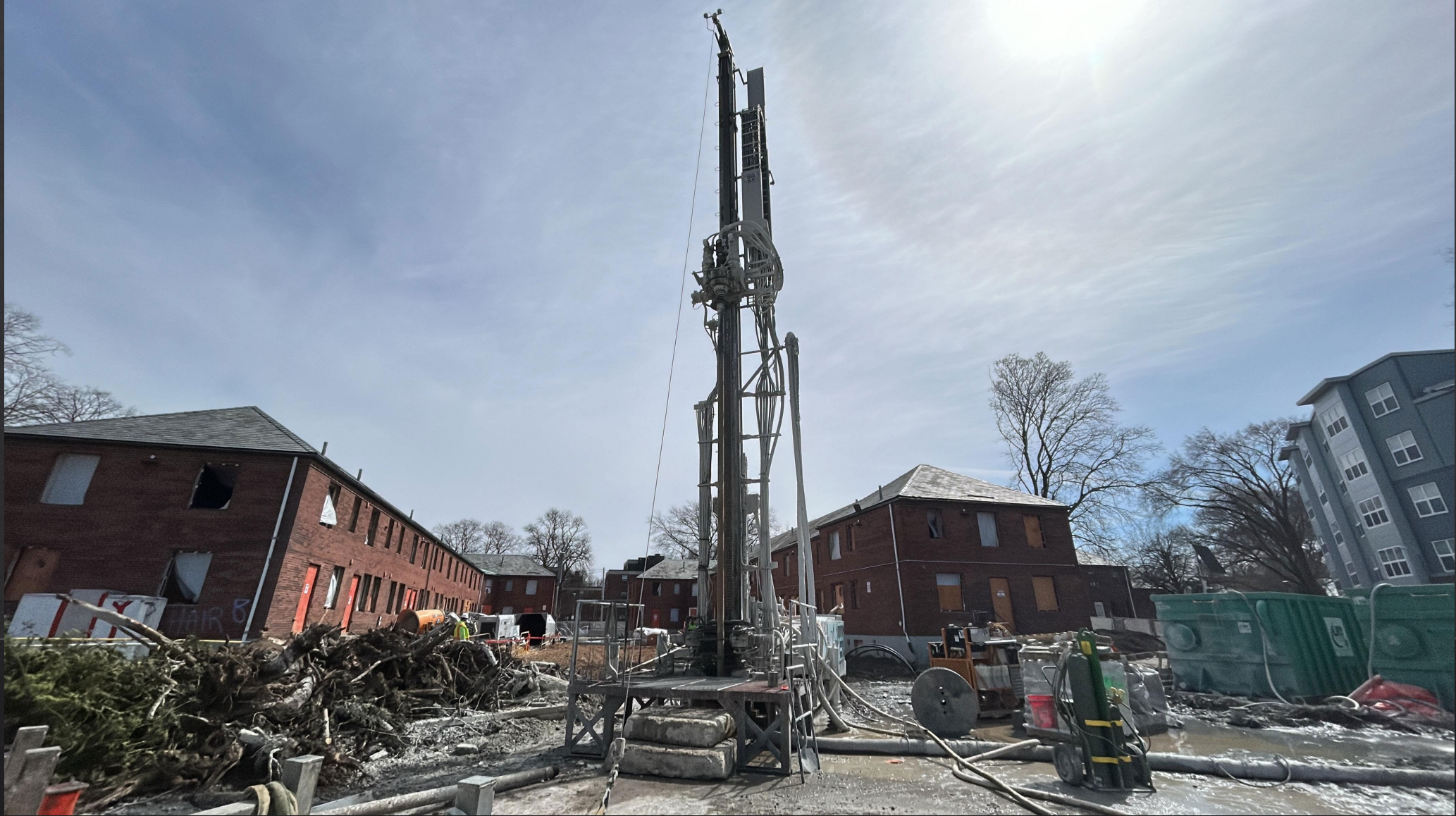
MEM – Building A – 22 Boreholes
