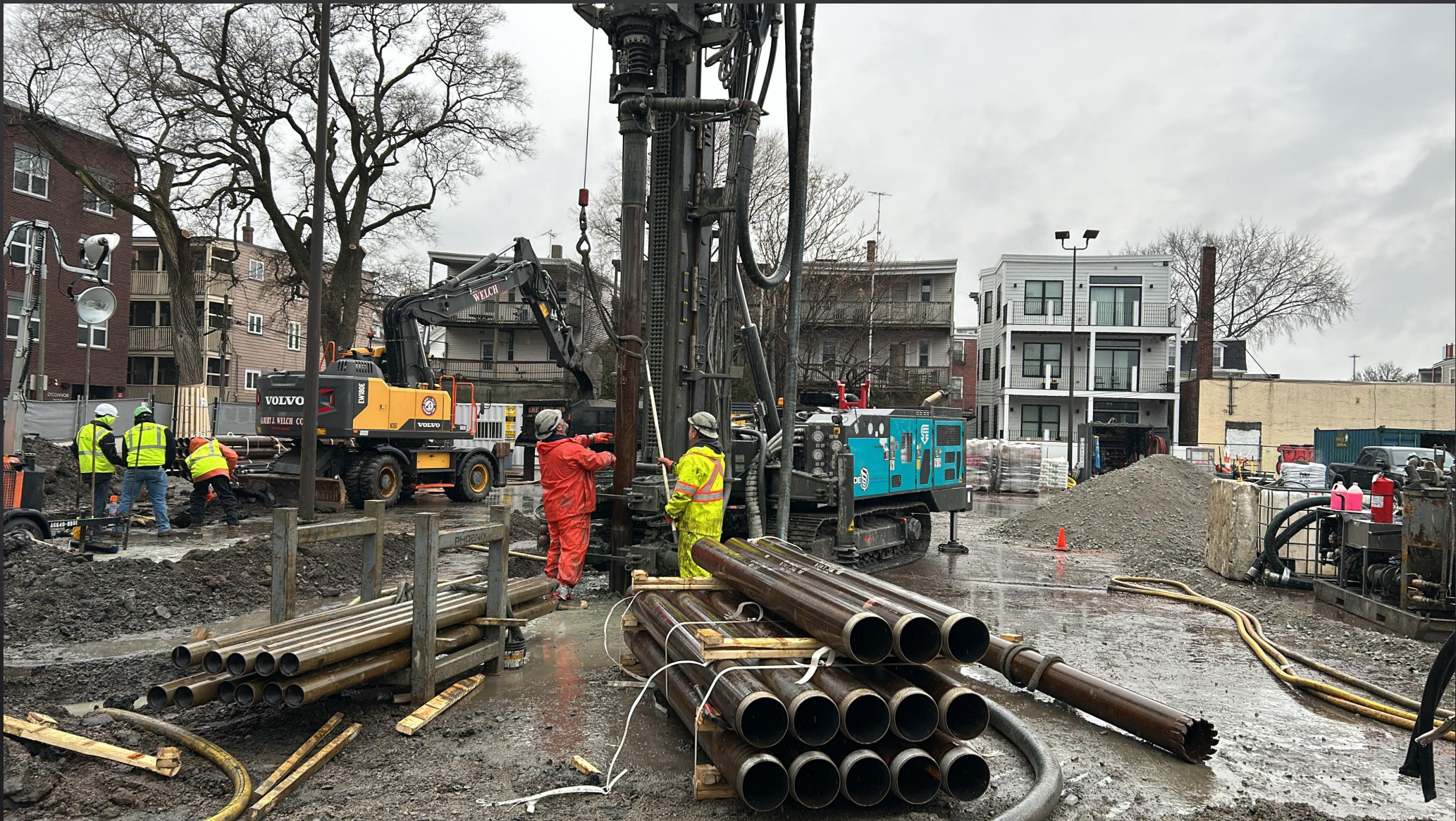
MEM – Building A – 22 Boreholes
