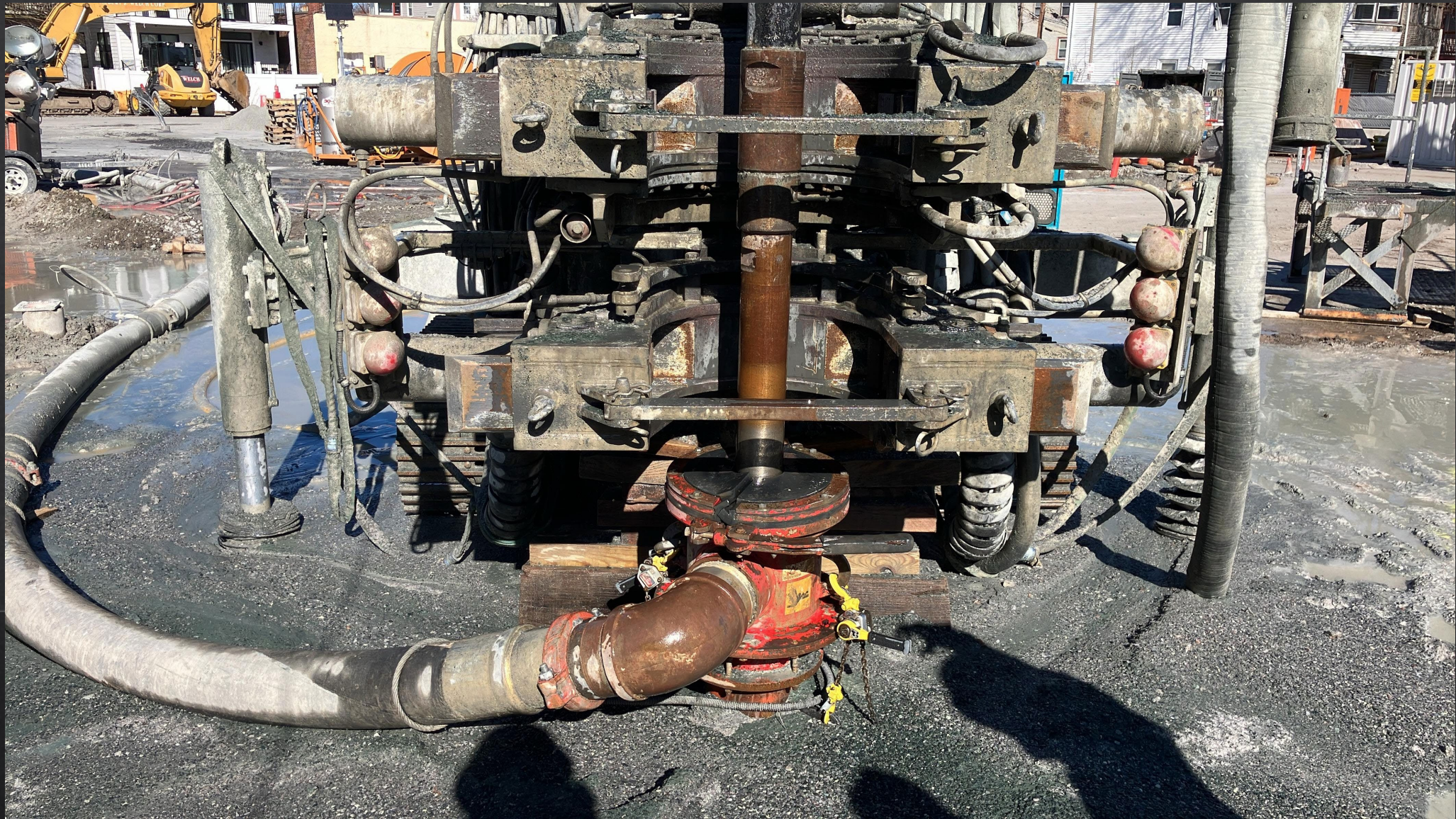
MEM – Building A – 22 Boreholes
