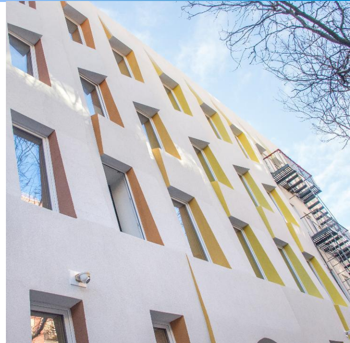
EIFS Façade with solar shading
