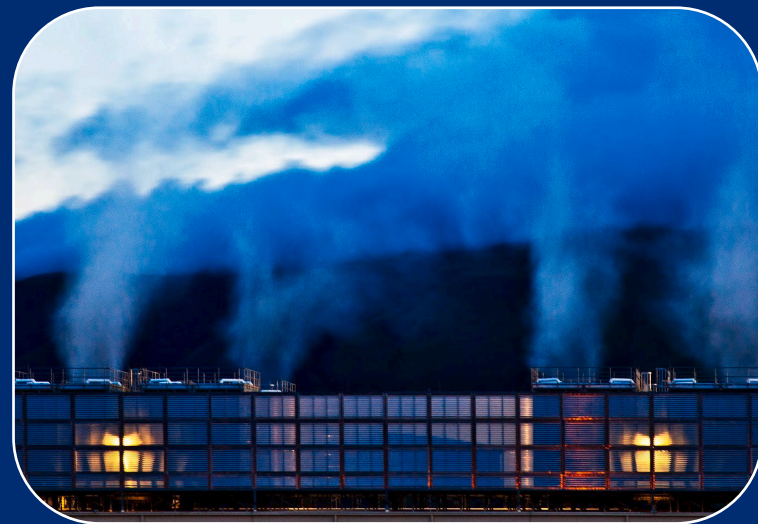
Data Center Heat Recovery
