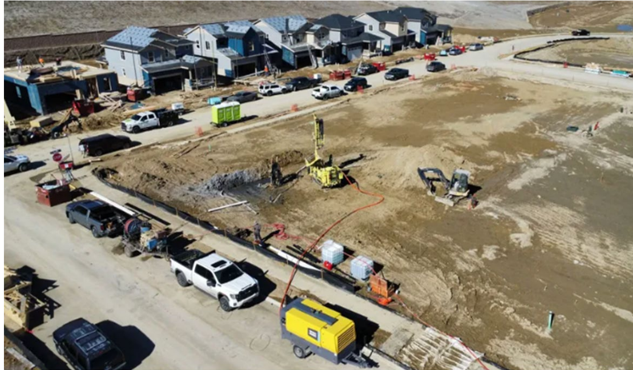
A drilling rig drills boreholes in the Ken-Caryl Ranch development in Littleton, Colorado. The boreholes are part of the Dandelion Energy geothermal ground-source heat pumps being integrated into newly built homes from Lennar. (Dandelion Energy)
